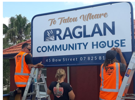
New Sign Install
